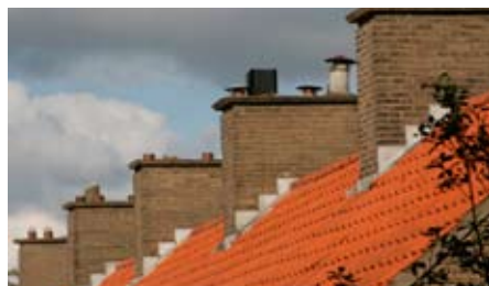
Household stoves and furnaces can constitute the primary source of surface air pollution
